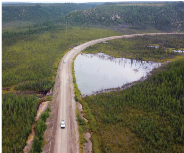
Figure 1. Part of the Dempster Highway north of Eagle River bridge, northern Yukon.
